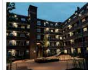
Figure 2. Rows of bulkhead lighting along these external walkways on the Shadwell Estate social housing estate in London have become a common element in the lighting of social housing. They are glory, crude and offer no optical control. The image above shows walkway lighting largely switched off versus, below, with it switched on. The contrast in terms of glare and light spill is significant, and telling. Photograph by Caterina Heckl
